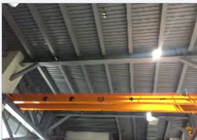
Daily energy saving indicator: illumination system
